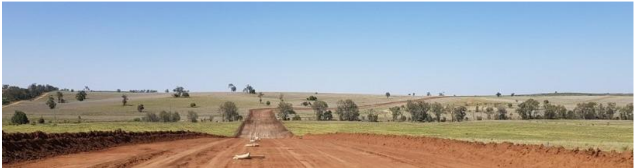
Plate 1: Typical construction RoW clear and grade
