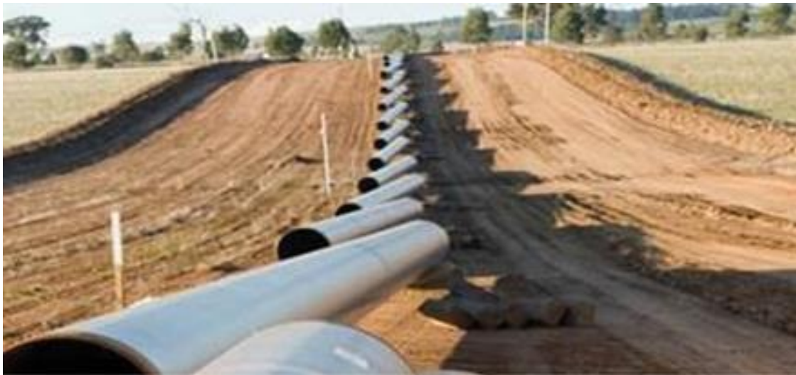
Plate 2: Stringing pipes
