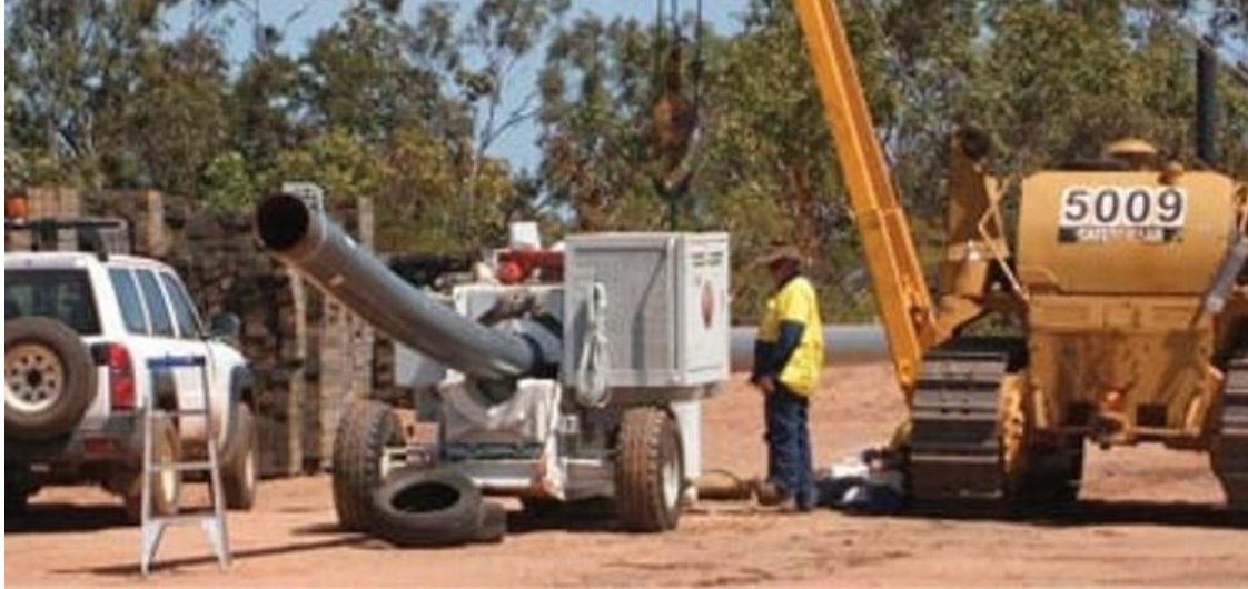
Plate 3: Pipe bending
