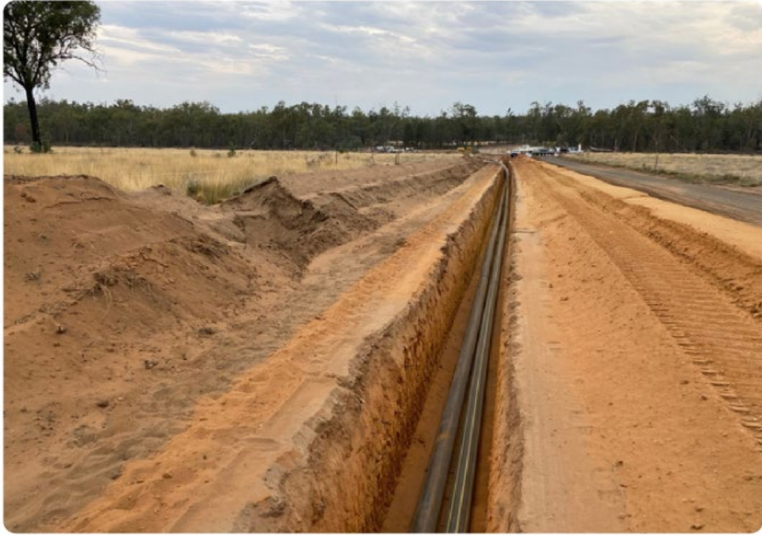
Photograph 2-1: Right of way at pipe installation stage showing temporary disturbance
