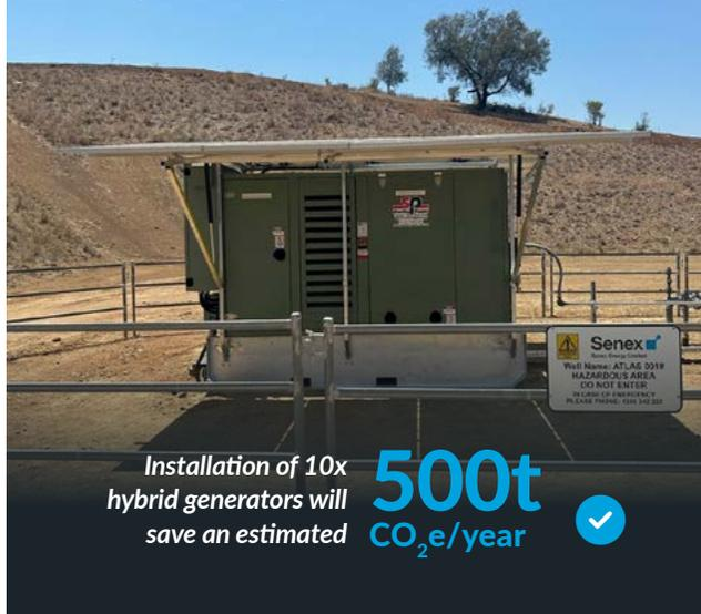
During the year, we moved from a field trial of solar and gas-fired generators to power our natural gas wells to manufacturing a fleet of ten at Australian-owned Shellby Power’s Brisbane factory.
